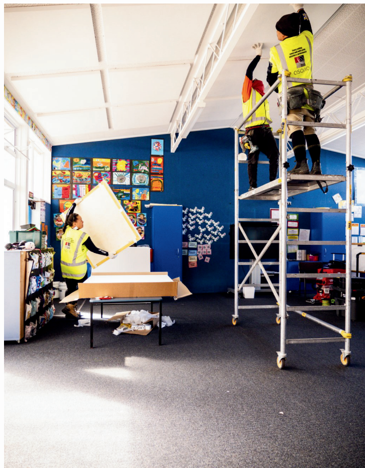
Triton CloudVG SIB installation
