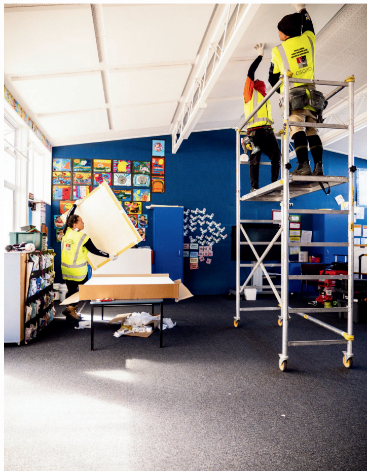
Triton CloudVG SIB installation
