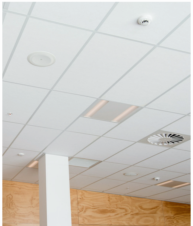
Photo: Triton 50HD, 600 x 1200 panels in Rondo Donn® grid
